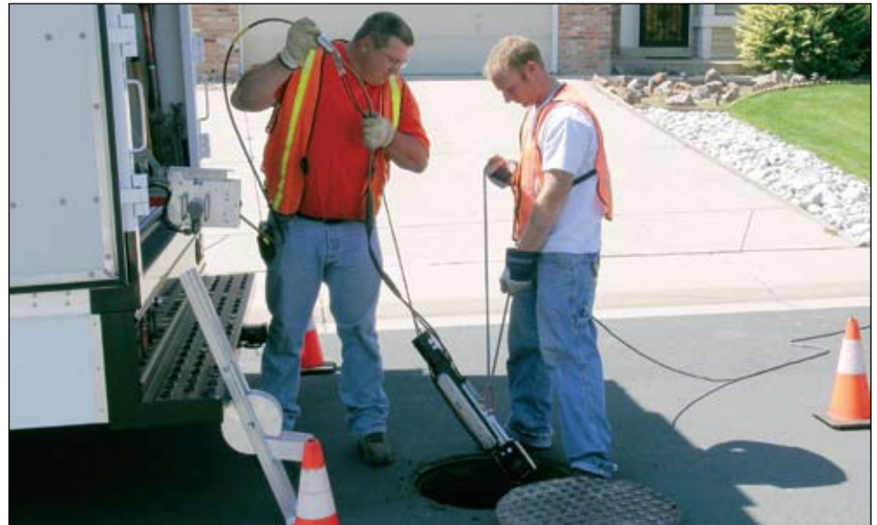
Platte Canyon will be using its sophisticated equipment to maintain sewer lines for Valley Sanitation District under a new agreement.
